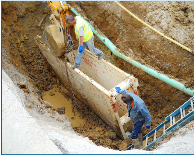
Work in progress on Gallaher Road to extend a section of the sewer line.
