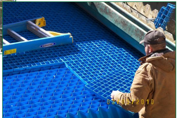
Ed Roberts is pictured on the right placing new tube settlers.
