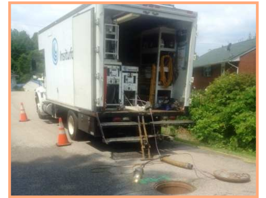
Annual visit from Insituform clearing and curing sewer lines.
