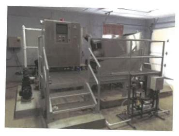
The Volute Dewatering Press is in and operating. The startup was completed on January 19 and we were able to fill two dumpsters by the end of the month. The 2 hauls to the landfill totaled 23.21 tons. This press is very user friendly and gives detailed information regarding the amount of polymer used, total gallons of liquid pressed, flow rate and polymer percentage rate.
