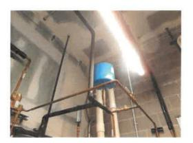
(The expansion tank should have a clamp similar to a riser clamp on it with 2 all thread rods supporting it)
