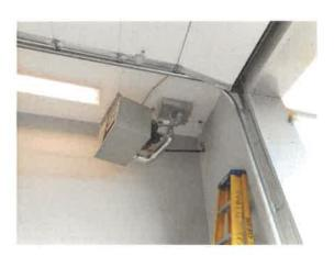
25. MECHANICAL 115 – TAPE THE RAW EDGE OF THE INSULATION AT THE BASE OF THE UNIT AND TAPE ANY TEARS IN THE DUCT INSULATION.
