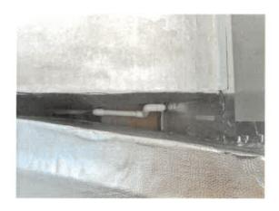
3. COVER ALL REFRIGERANT PIPES OUTSIDE THE BUILDING WITH ALUMAGUARD OR ALUMINUM JACKET PER SECTION 230700, 2.1 AND THE DETAIL ON M2.1.
