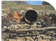
STORMWATER CULVERT THAT DUMPS IN RIVER
